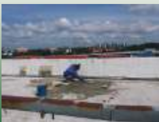
Teson Slurry Flex TW-151 Crack Line Repair
